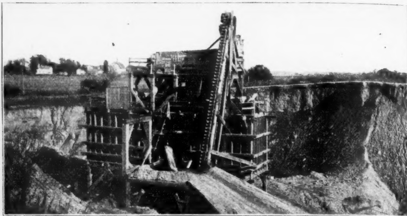
The Initial Grizzly, Crusher and Bin.
